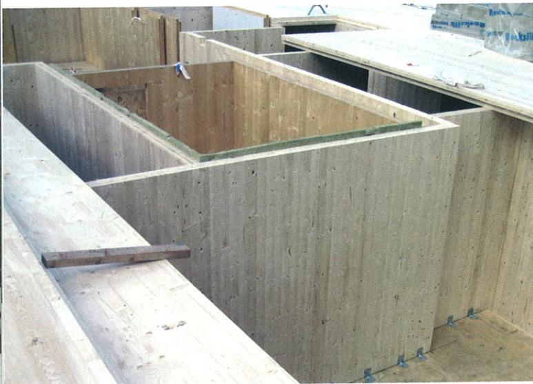
Clockwise from right Murray Grove; Fifth-floor plan; Wall section; Construction view of cross-laminated panels secured with steel angle brackets
