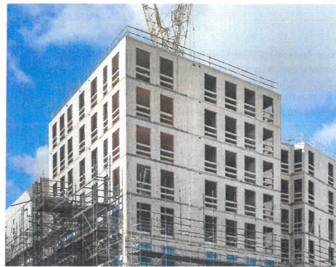
Mid-rise wooden buildings – these are in London – can be put together in a few days
